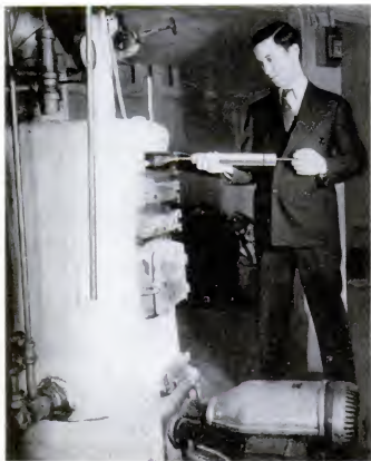
Sprayed into the furnace, the compound removes soot
